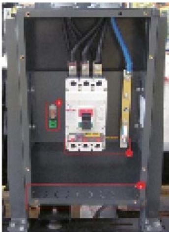
Figure 3.2 Gen-set field wiring of load cables
